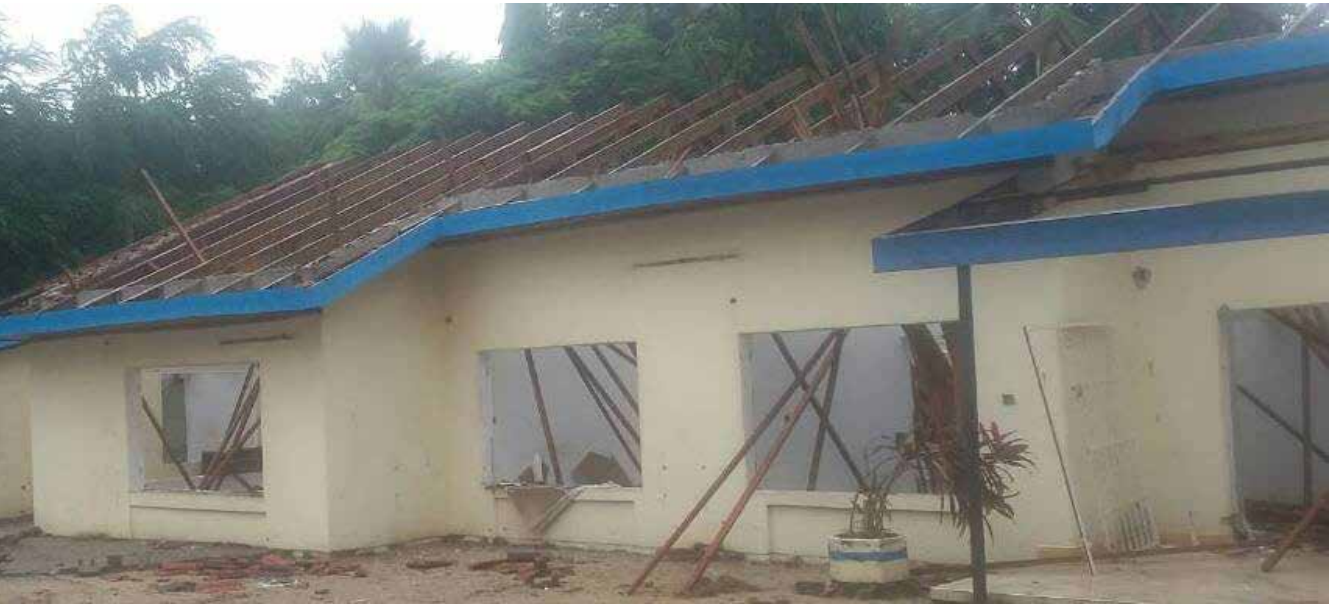
Demolition of TLS House on plot 391
