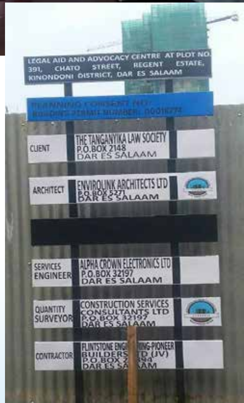
Sign board evidencing construction commencement
