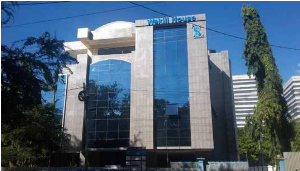
LAAC Building at its final stage
