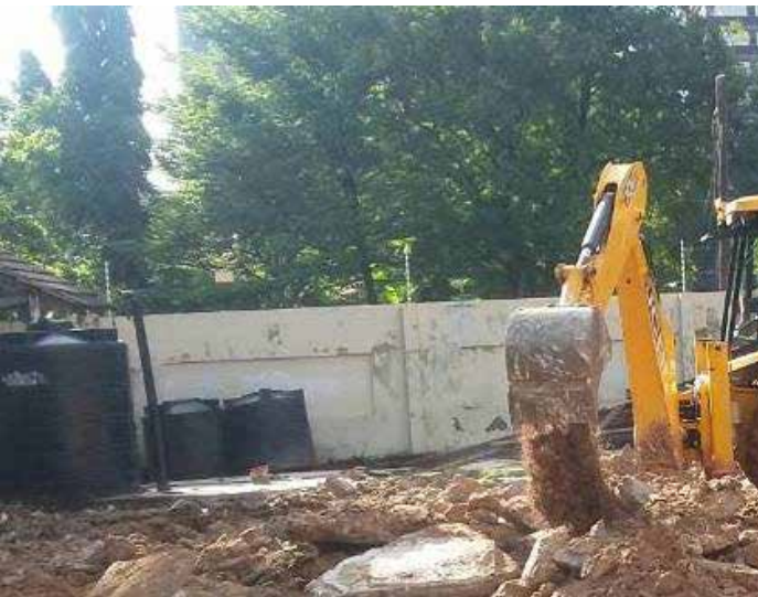
Figure 3 Site clearing after demolition
